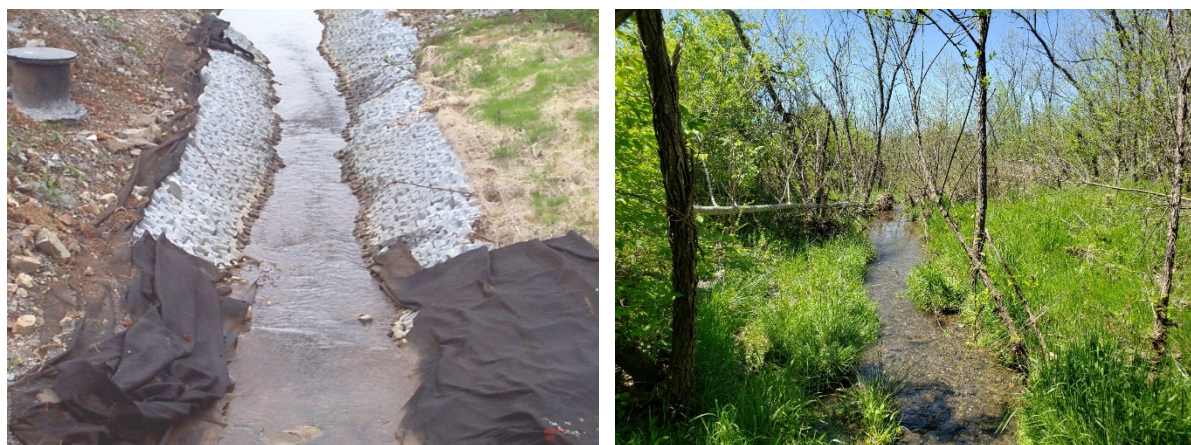
Figure 3.50. Construction of lined section of Mitchell Branch, MIK 0.7, in 1998 (left) and more recent habitat conditions in 2019 (right)
